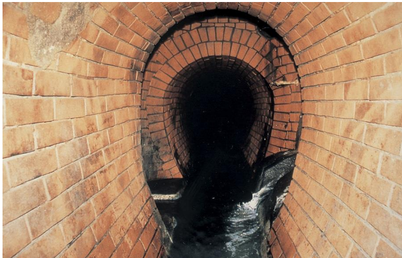
Figure 1 First Modern Sewer Installed in 1884, still used, Kanda, Tokyo
