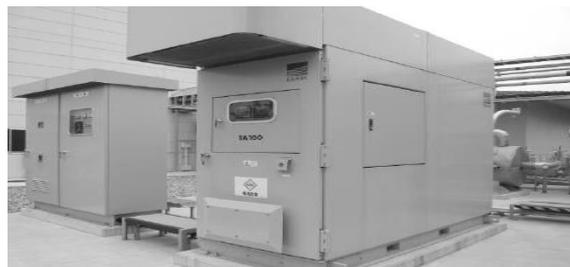
**Figure 12 Micro Gas Turbine**
