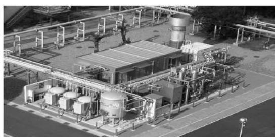
Figure 8 Purification and Injection Facility for City Gas Use
